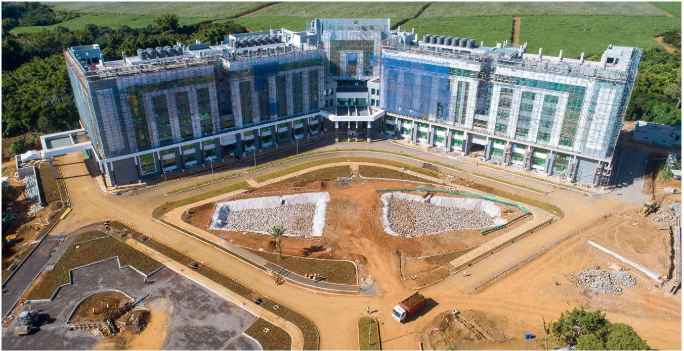
Construction of teaching Hospital at Flacq, Mauritius
